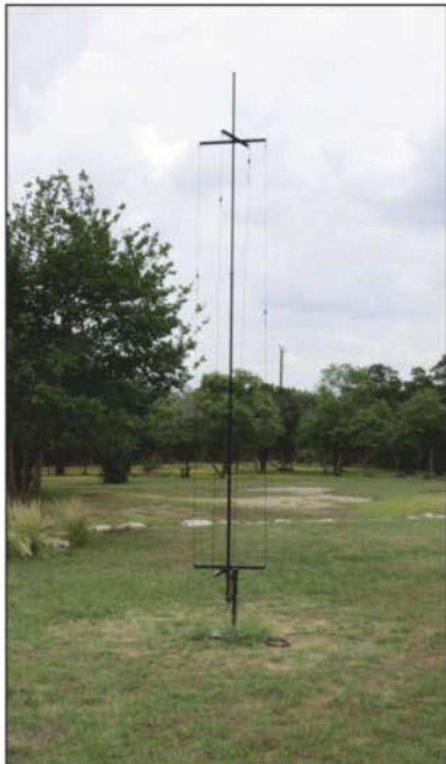
Photo A. The Texas Star is a 5-band vertical that requires no tuner and has a single feedline. The central antenna element (a COMTEK COM-20VA 20-meter vertical) supports two sets of cross-arms for additional band elements. (All photos and drawings courtesy of the author)
