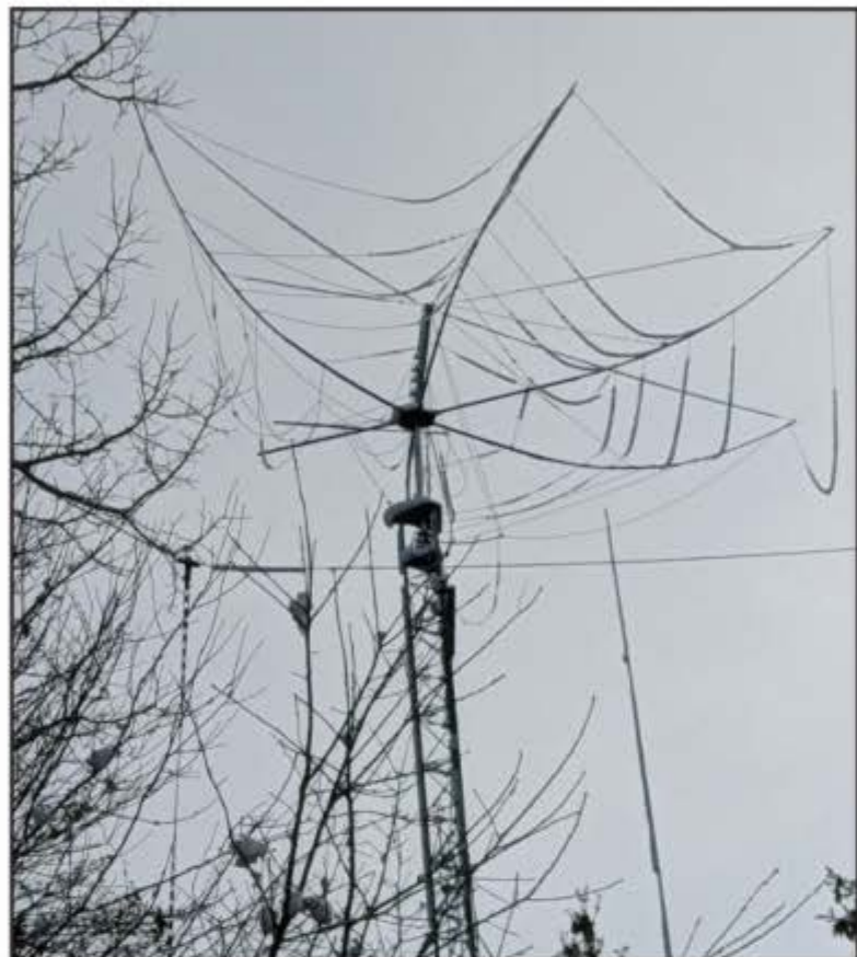
Photo B. K1GUY's prior hex beam after ice storm.
